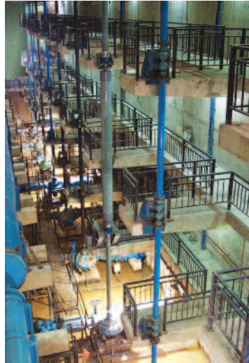
A 3-section Form-Flex Composite vertical driveshaft (gray, in center) was used to replace both the 4-section shafts originally installed (blue, in foreground, on right) and the 4-section U-joints (black, in background, on left).
